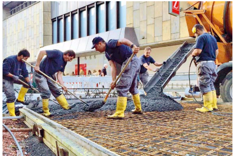
Abb. 9: Betonage
